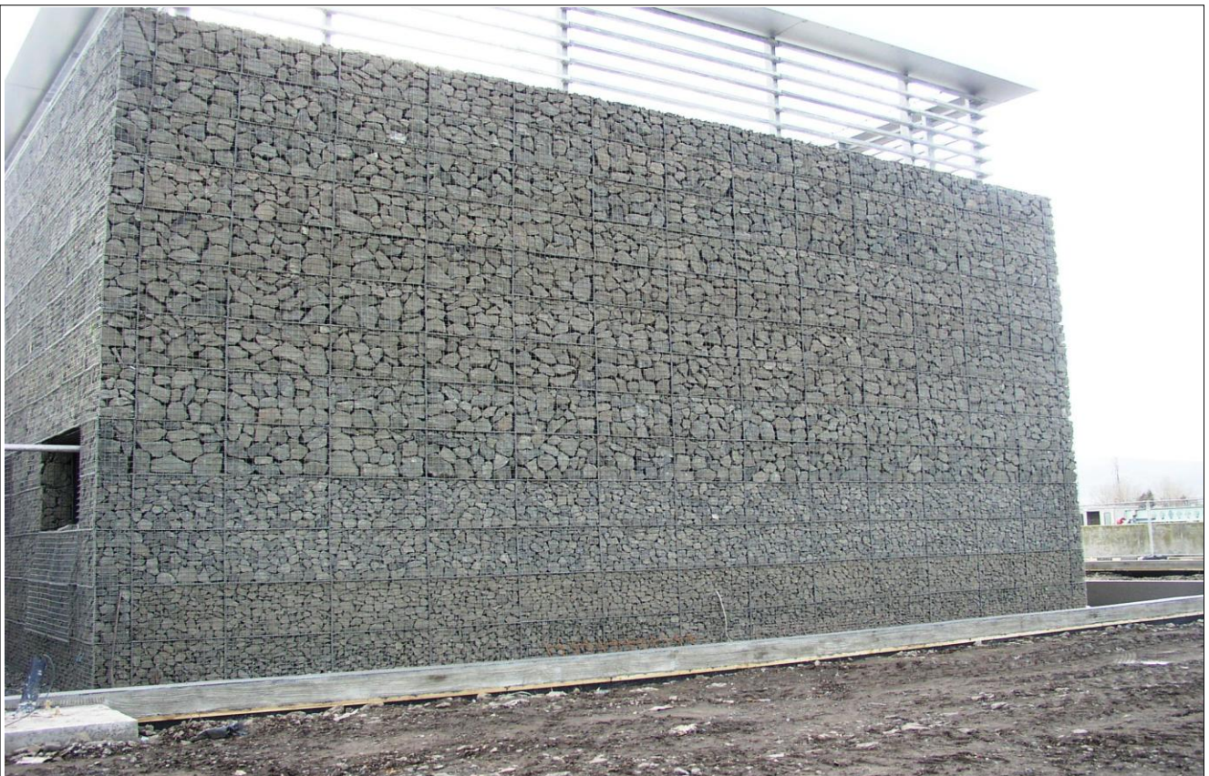
ARCHITECTURAL PROJECTS DEMAND CONSIDERED SELECTION AND PLACEMENT OF THE STONE
