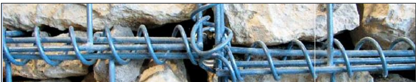
CORNER JUNCTION AT FOUR ADJACENT GABIONS SHOWING SPIRALS AND LOCKING PINS TO CONSTRUCT A STRONG MONOLITHIC STRUCTURE
