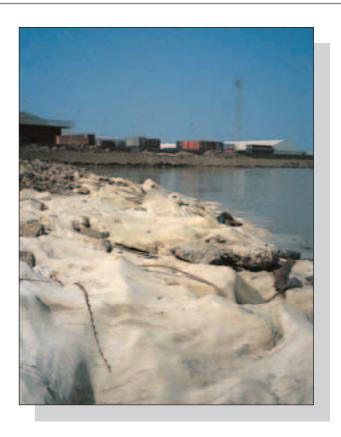
impermeable clay closure bund (to 5.0 m A.O.D.) across the mouth of the basin. On completion of the closure bund a number of smaller bunds (to 1.5m E.G.L.) are constructed within the basin forming a series of cells. The filling of the cell areas is undertaken using general excavated material in 0.25 m thick layers with the finished ground level being reached at 5.0 m A.O.D.
