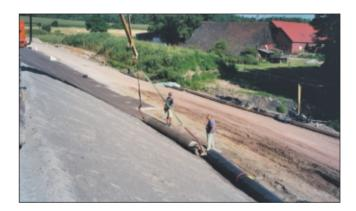
was used to encapsulate the tailings material (i.e. coal spoil) and avoid water penetration even during flooding.
