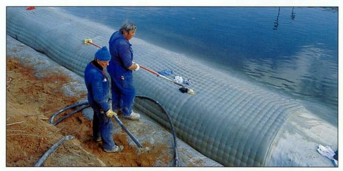
water from the fill material. Incomat® concrete mattresses can be installed above and below water (up to depths of 50 m) and can cope with flow velocities up to 2 m/s.
