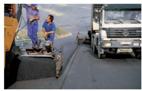
HaTelit® C is a flexible polyester grid incorporating an ultra-light nonwoven, also bitumen coated, which is applied to prevent reflective cracking.
