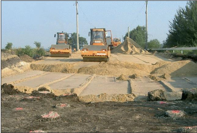
*Cut off vibro columns in piled foundation and incorporation of mixed aggregate layer*
