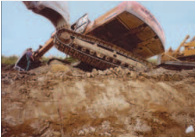
Result of an active sinkhole
