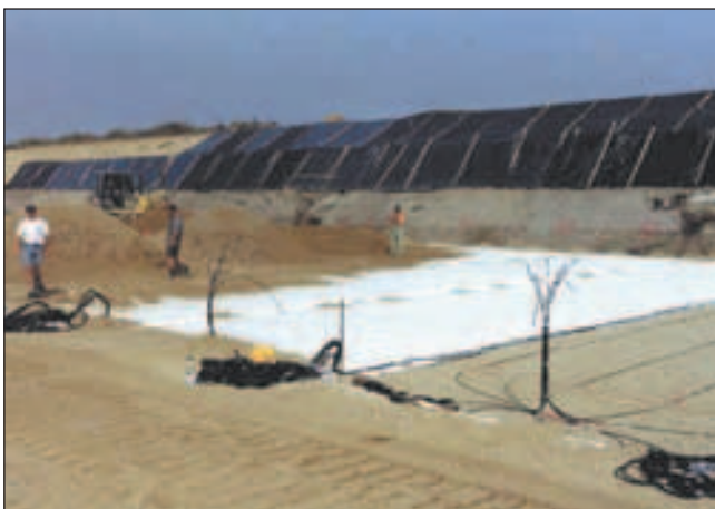
Installation of warning layer and monitoring system
