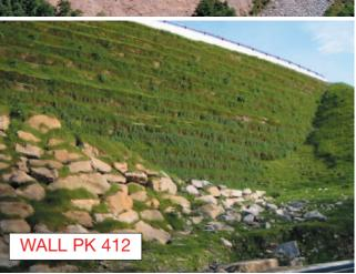
gravel layers, reinforced with **Fortrac**<sup>®</sup>. This geogrid is made from high tenacity polyester yarn with strength from 110 to 150 kN/m<sup>2</sup> and a special mesh size of 50 x 50 mm. This generously-sized mesh facilitates better interlocking between this type of backfill and the geogrid.
