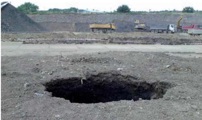
Fig. 6: Sinkhole forming during construction
