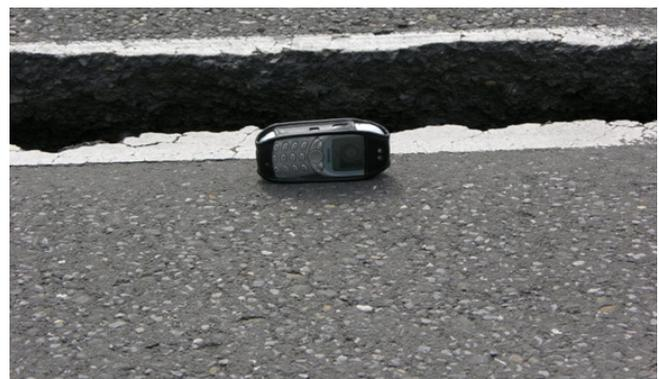
Fig. 5: Deformations forming differential movements, DK 44 Poland
