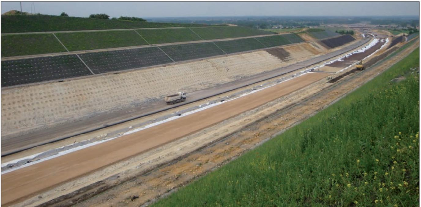
Fig. 13: Fortrac 3D® slope reinforcement in cut section
