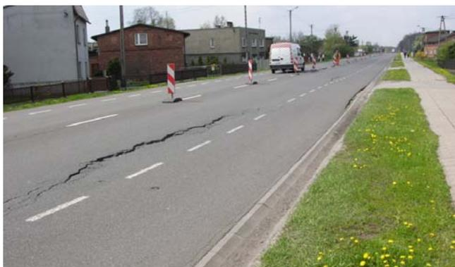
Fig. 4: Surface deformation due to mining activity, DK 44, Poland
