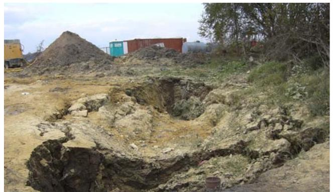
Fig. 7: Sinkhole forming during construction
