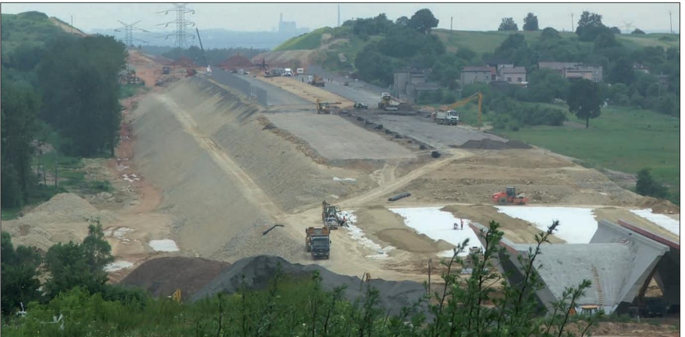
Fig. 15: Fill section of highway embankment
