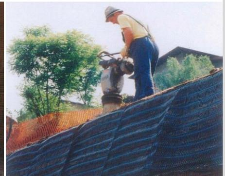
HAND / PLATE COMPACTING FIRST 1.0m FROM FACE
