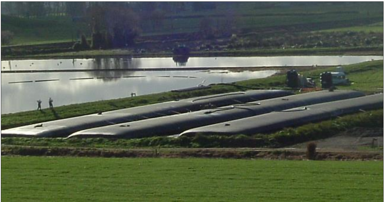
14 METRE CIRCUMFERENCE TUBES DEWATERING SLUDGE AT A MUNICIPAL SEWERAGE POND
