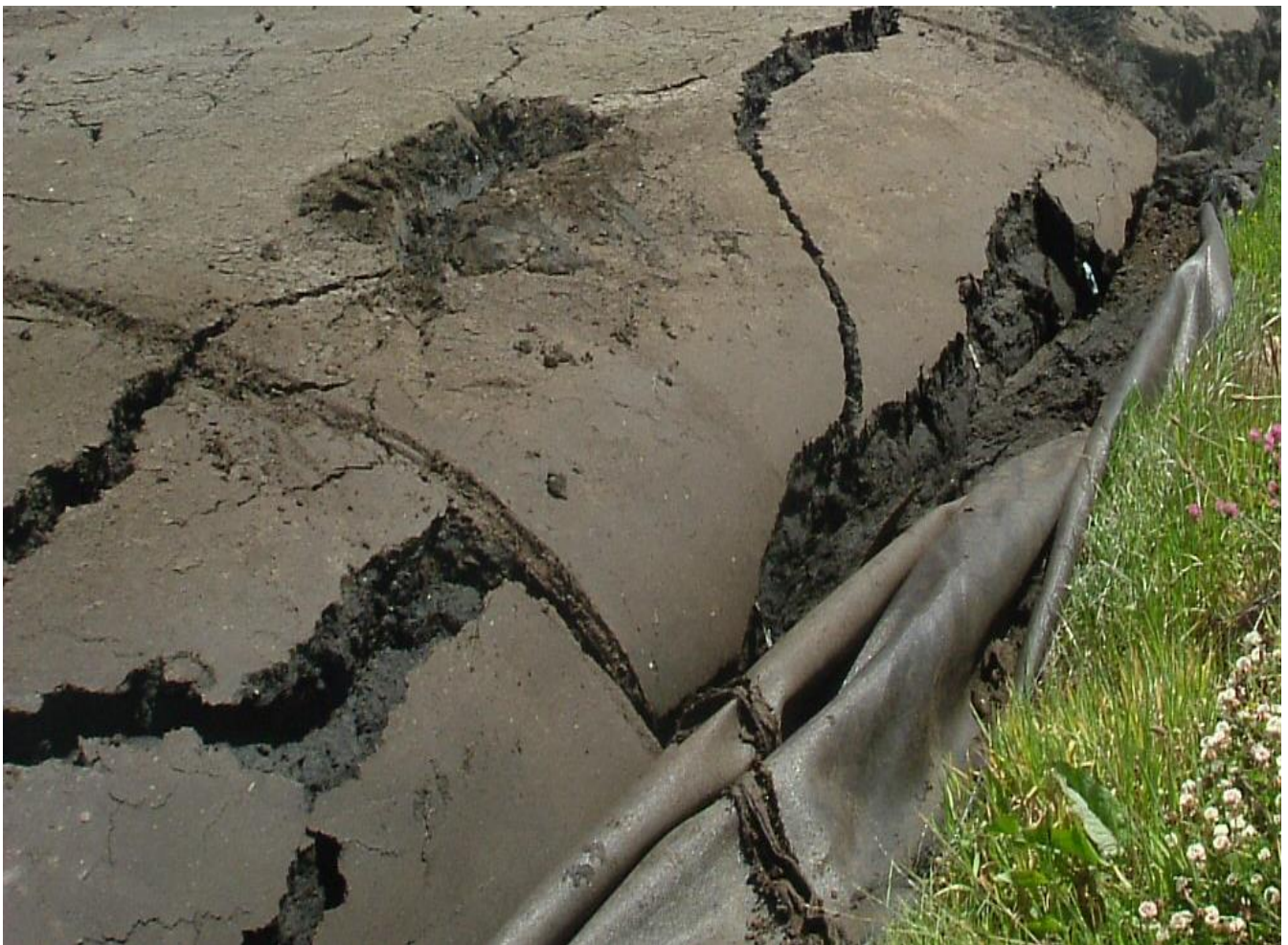
SOILTAIN® TUBE CUT OPEN AFTER COMPLETION OF DEWATERING DRY SLUDGE READY FOR DISPOSAL TO A LANDFILL
