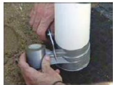
Seal base of pipe with adhesive tape and silicon.
