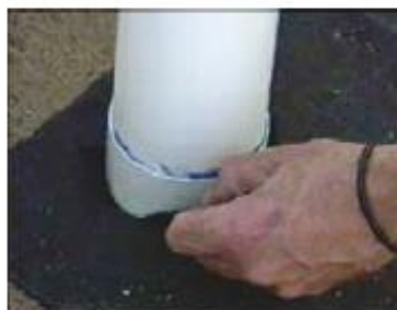
Slide the pipe through the geotextile and the hole made in the Atlantis module.
