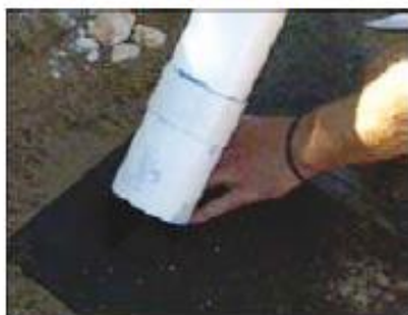
Place pipe into the X cut hole of the geotextile.
