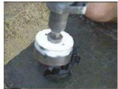
Core drill into the Atlantis module.
