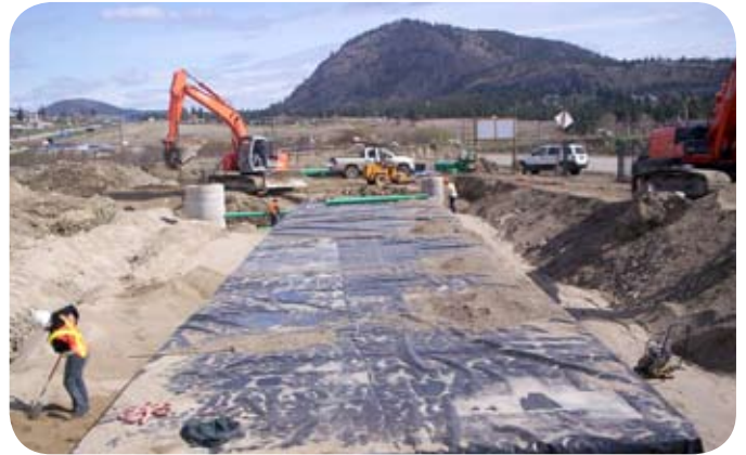
Backfilling the tank.
