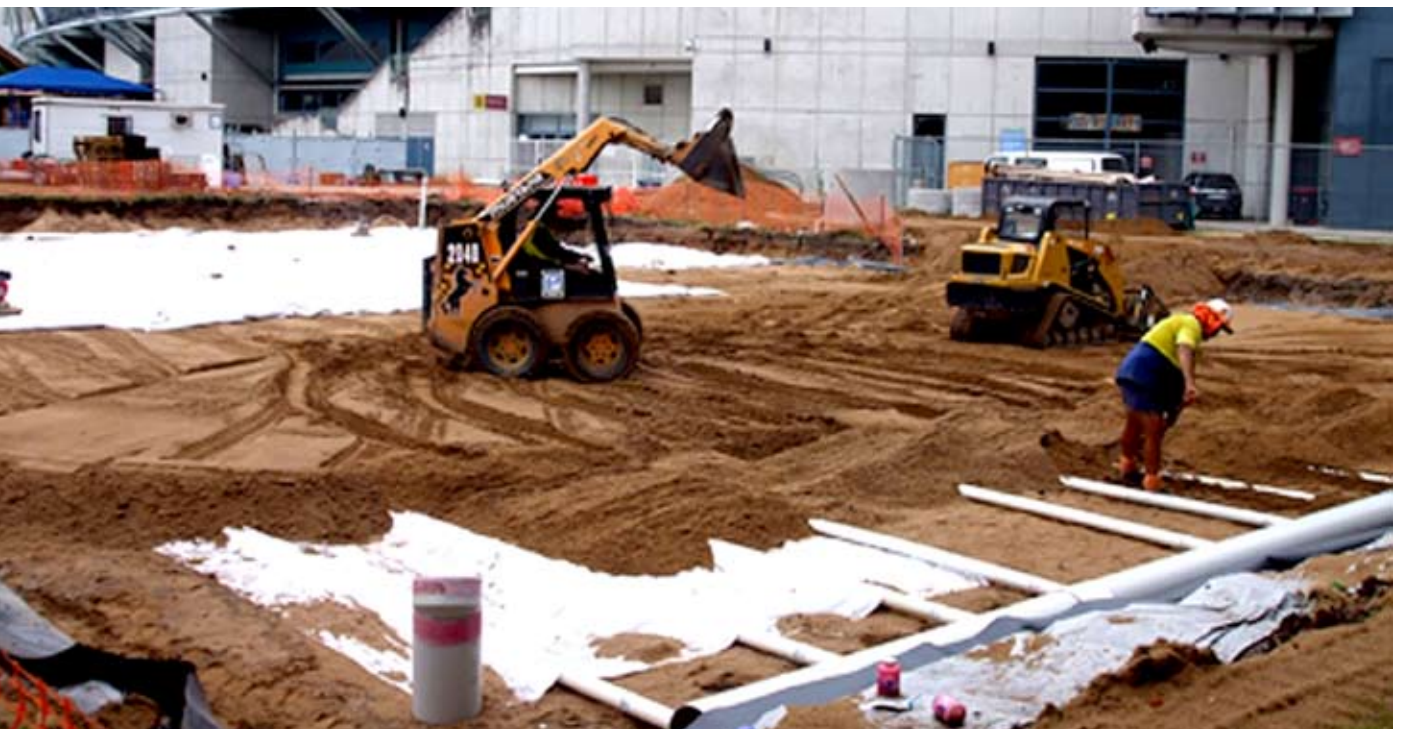
Downpipe dispersion and infiltration system.
