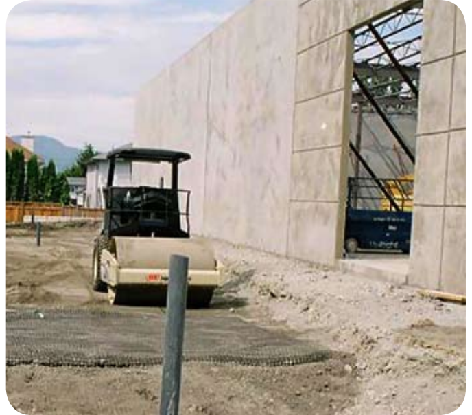
Adding Geogrid on top of the backfilled tank.
