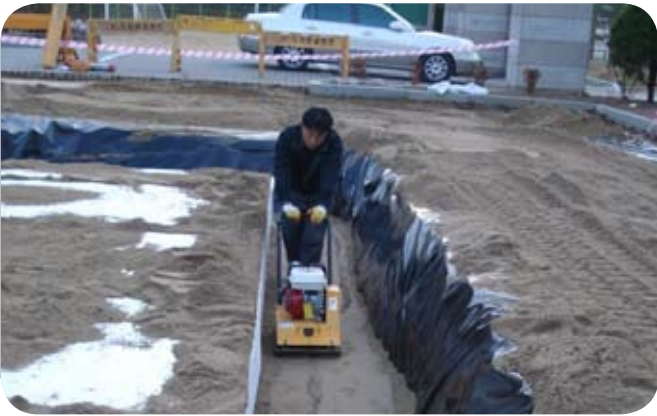
Backfilling the sides of the tank
