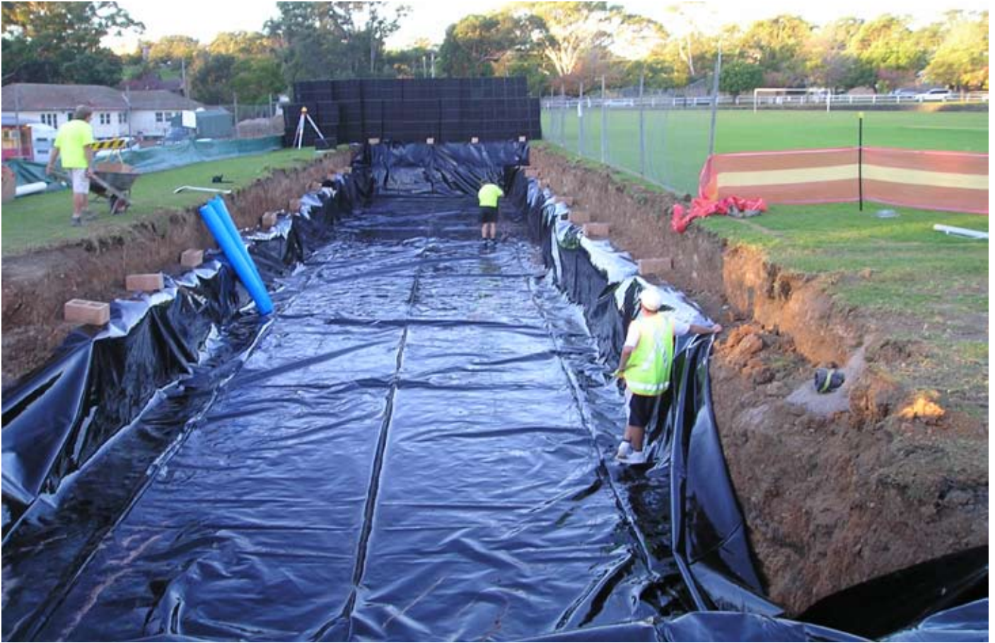
Laying of impermeable liner in the excavated area.
