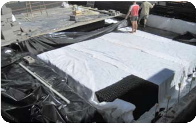
The Atlantis® Matrix® tank modules wrapped in Geotextile.
