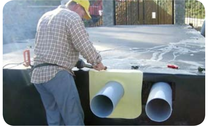
The tank fully wrapped in the first layer of impermeable liner.
