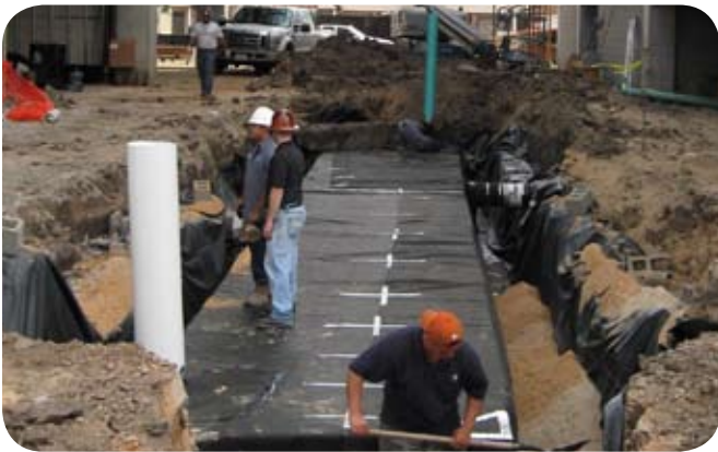
Backfilling the Atlantis® Matrix® (D-Raintank®) modules.
