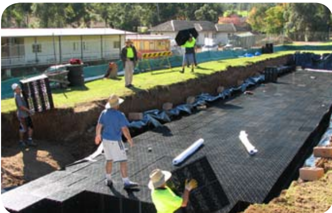
Installing the Atlantis® D-Raintank® (Matrix®) on top of the Geotextile.
