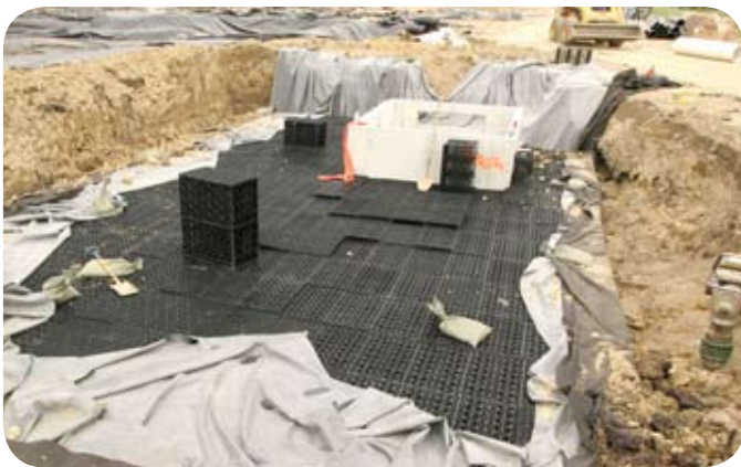
Tank Backfilling and water feature installation.
