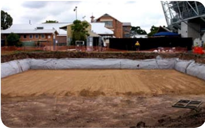
Prepared base of sand for level installation of modules.
