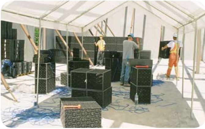
Assembling the Atlantis® D-Raintank® (Matrix®) boxes.
