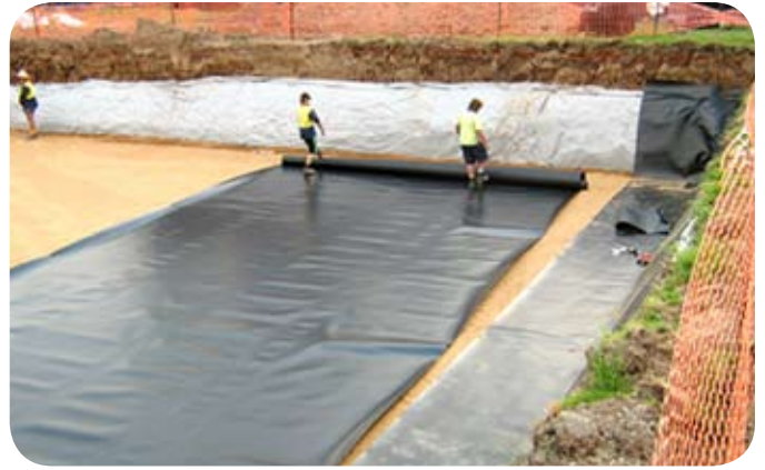
Rolling out the Geotextile and the Waterproof Liner.
