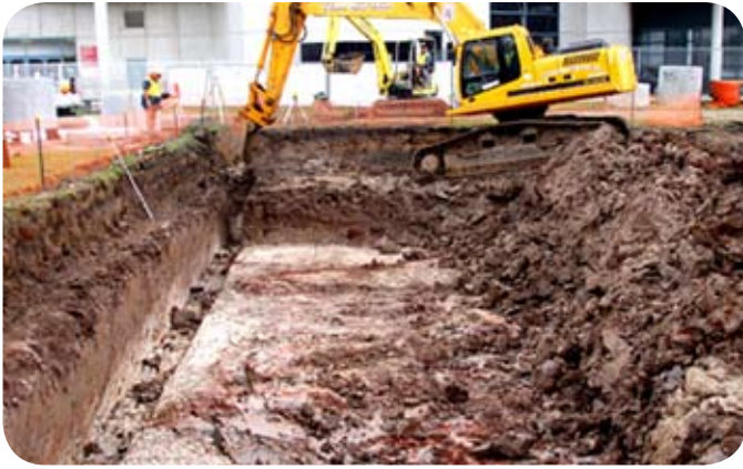
Preparing the excavation for the Matrix® tank installation.
