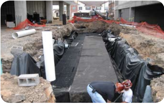
Wrapping the Atlantis® Matrix® (D-Raintank®) modules in Geotextile.
