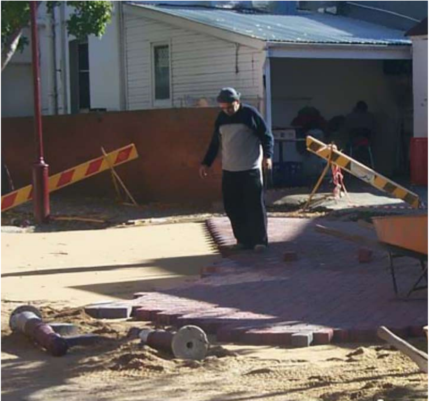
Installation of interlocking permeable paving.
