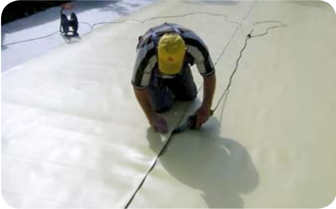
Welding the first layer of impermeable liner.
