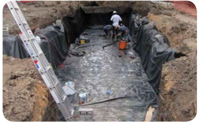
Installed Liner.
