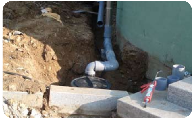
Atlantis® Filtration Unit installed in place.
