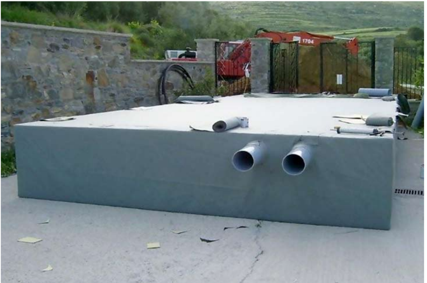
The tank wrapped in the second layer of impermeable liner.
