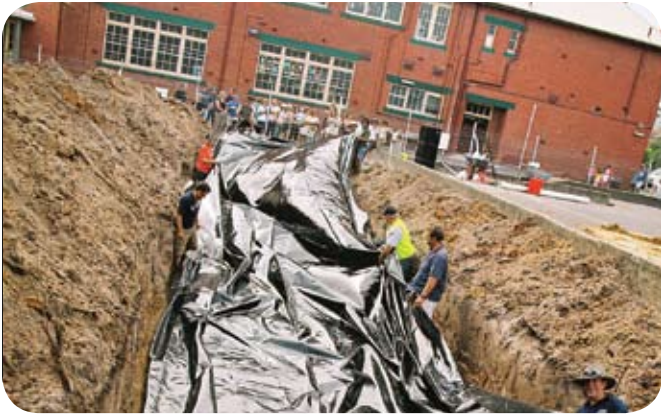
Laying of impermeable liner for re-use systems.
