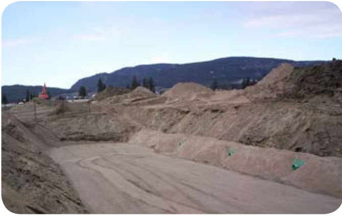
Excavation preparation and levelling for the Atlantis® D-Raintank® (Matrix®) System.
