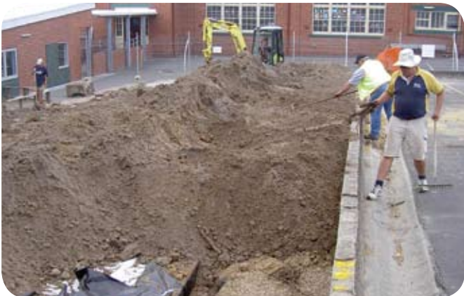
The backfilled tank ready for soft fall landscaping.
