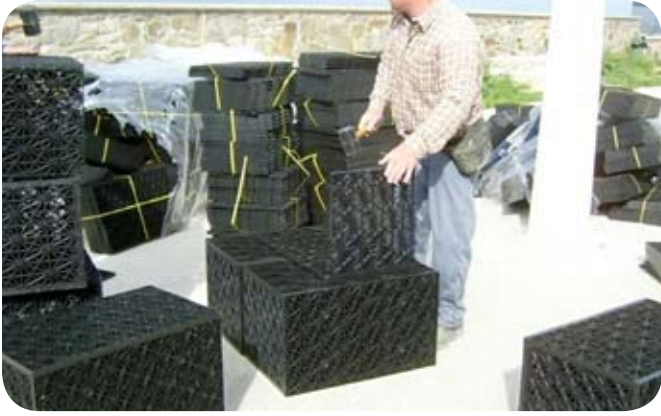
Assembling the Atlantis® Matrix® (D-Raintank®) modules.
