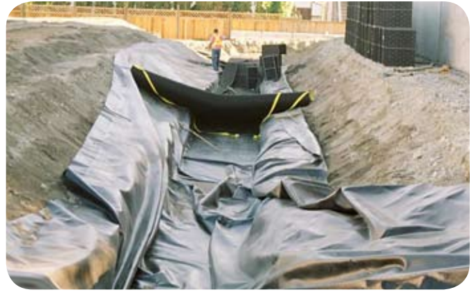
Atlantis® D-Raintank® (Matrix®) modules wrapped in geotextile, waiting to be further wrapped in impermeable liner.
