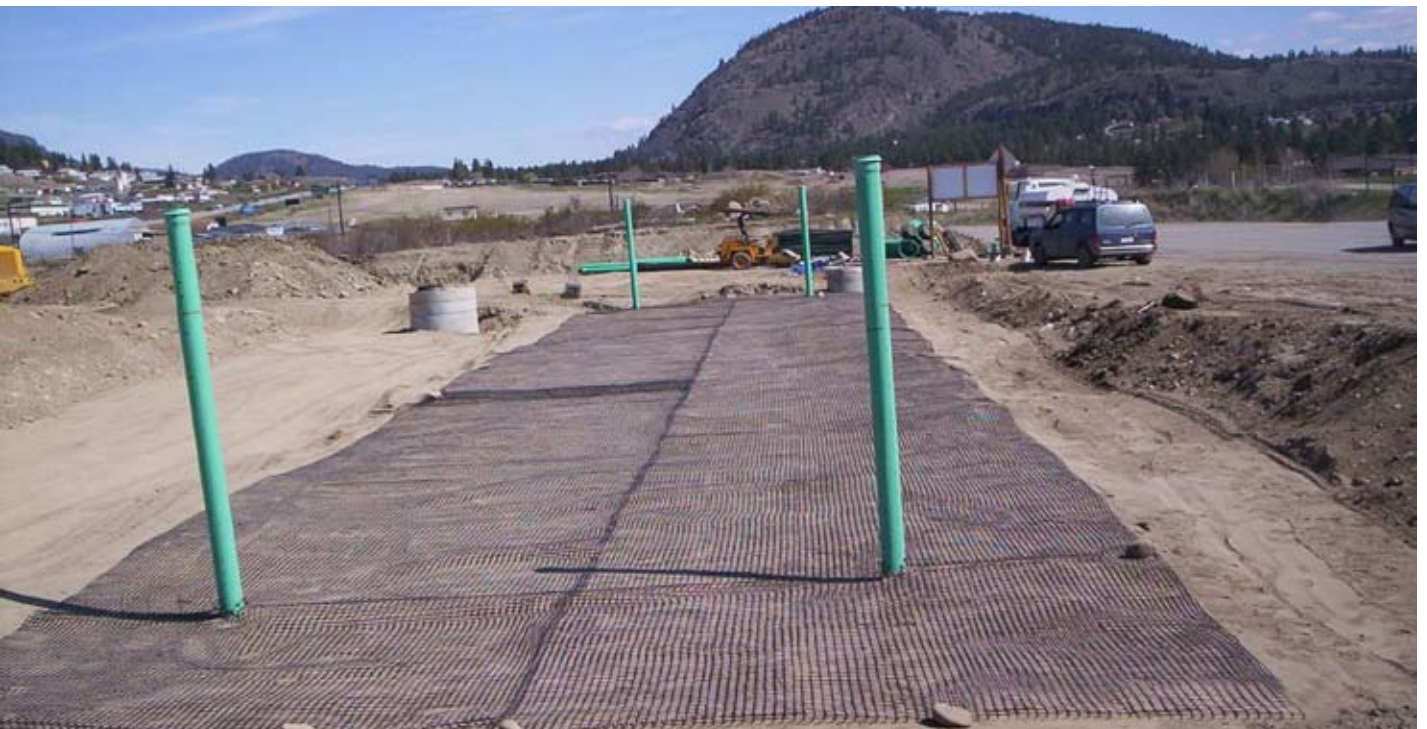
Adding Geogrid on top of the backfilled tank.
