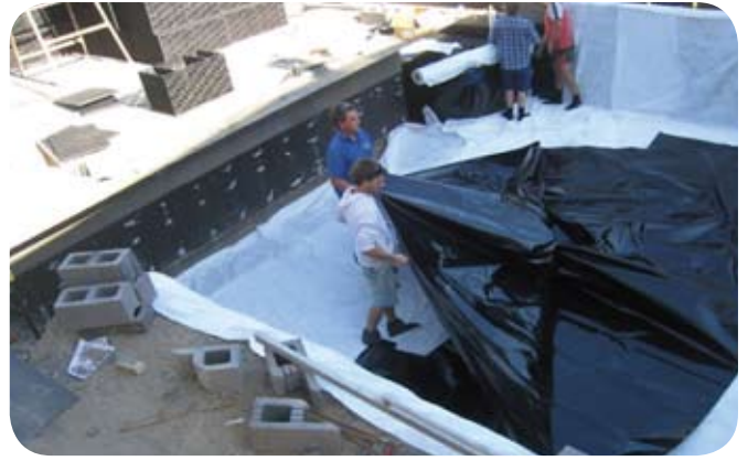
Installing the geotextile and the impermeable liner.
