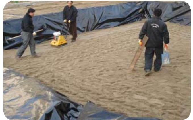
Backfilling the top of the tank
