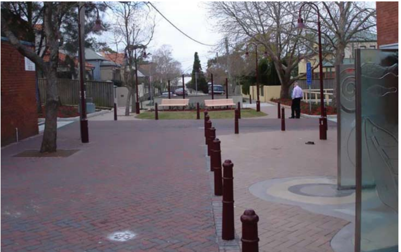
Looking west across the permeable paving threshold between the two carpark areas.
