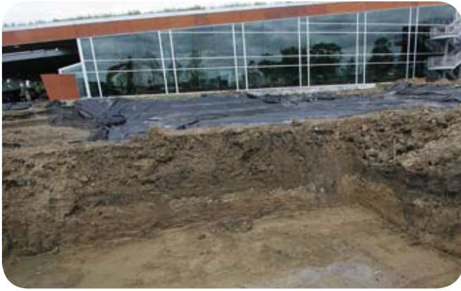
Excavation preparation for the Atlantis® D-Raintank® (Matrix®) System.
