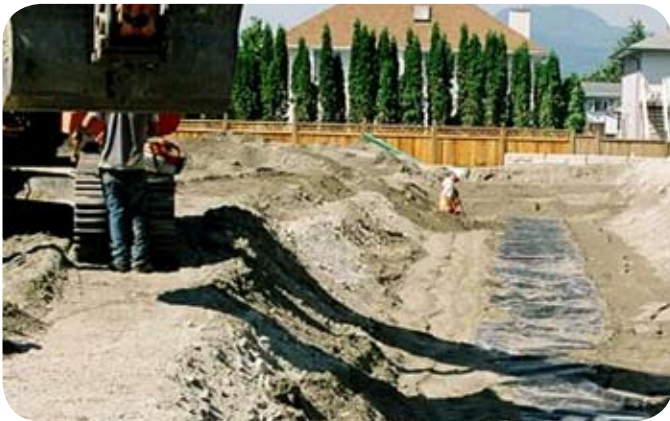
Backfilling the tank.
