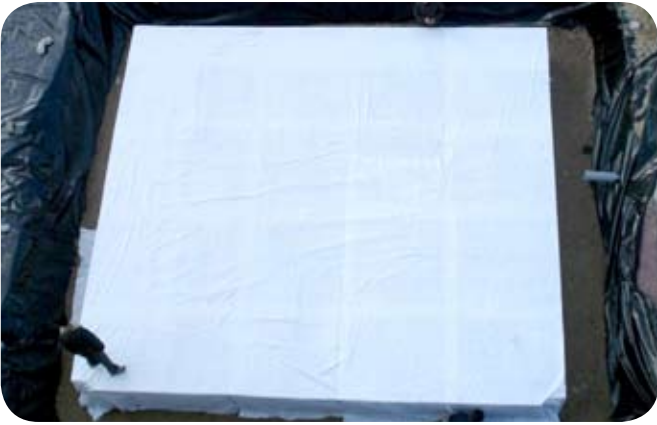
Tank modules wrapped in geotextile laid on top of the plastic liner.
