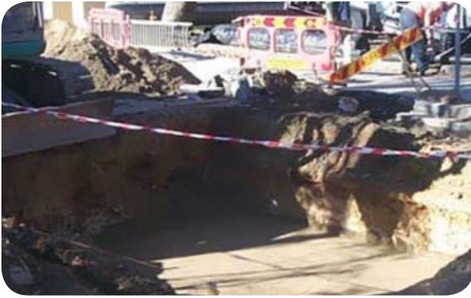
Excavation for water tank. Note bedrock at bottom of excavation.
