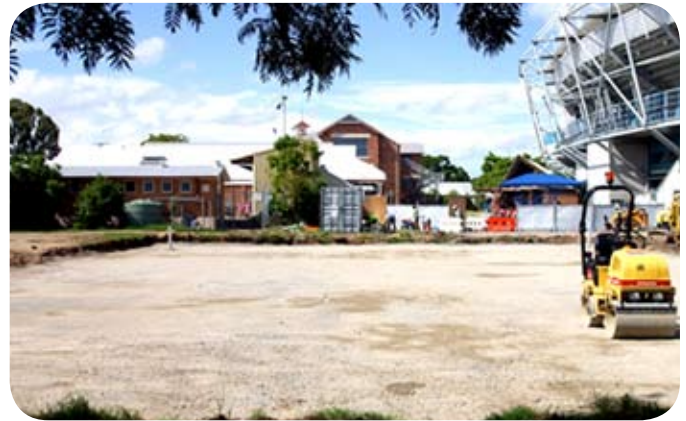
Installation ready for last layer of compacted backfill.
