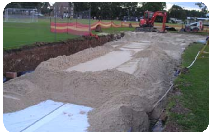
Backfilling the tank.
