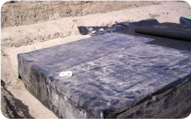
Atlantis® D-Raintank® (Matrix®) modules wrapped in impermeable liner.
