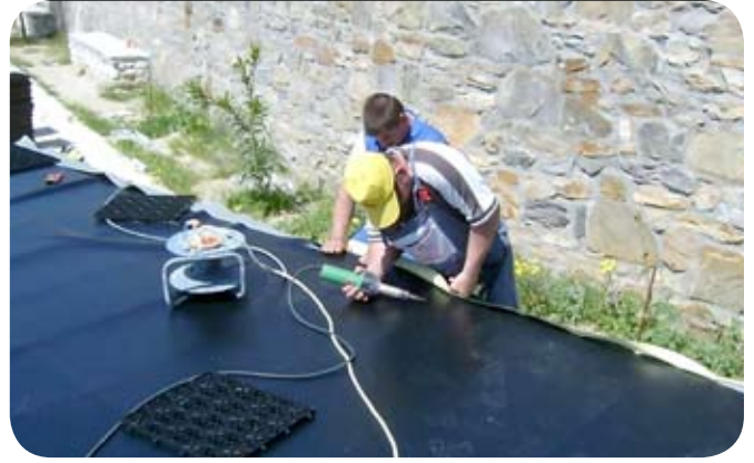
For extra protection an additional layer of impermeable liner was installed.
