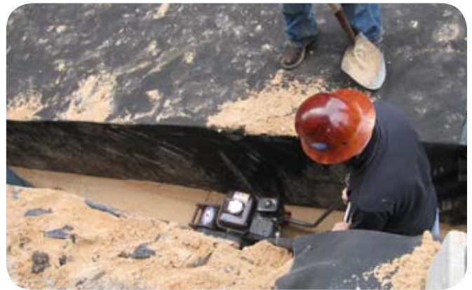
Backfilling the sides of the tank.
