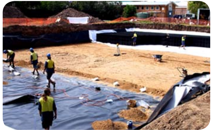
Ecological sand treatment layer being prepared.
