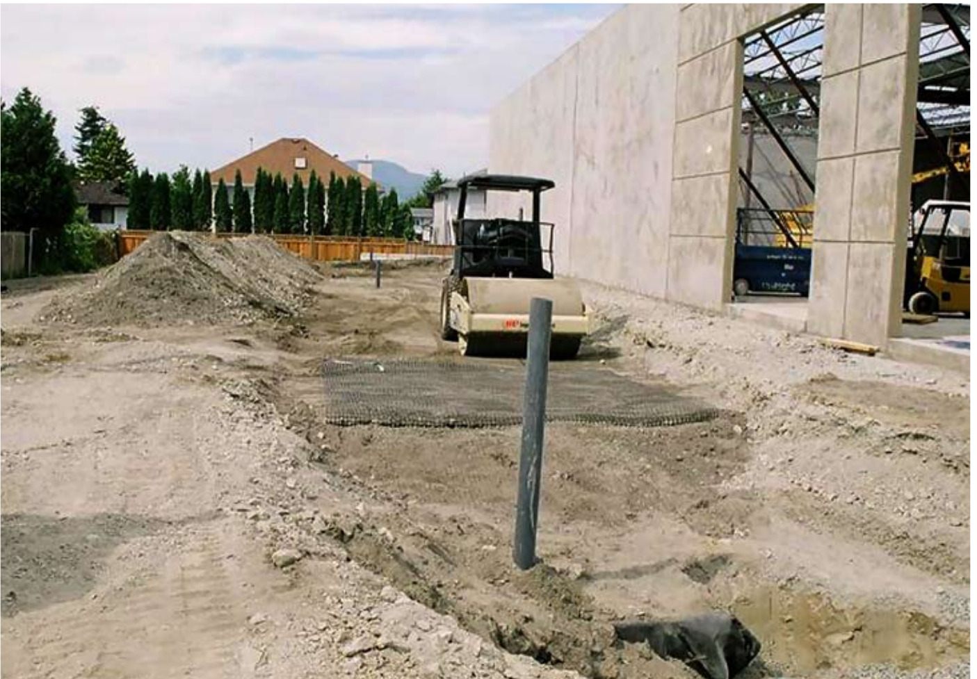
Backfilling the tank.
