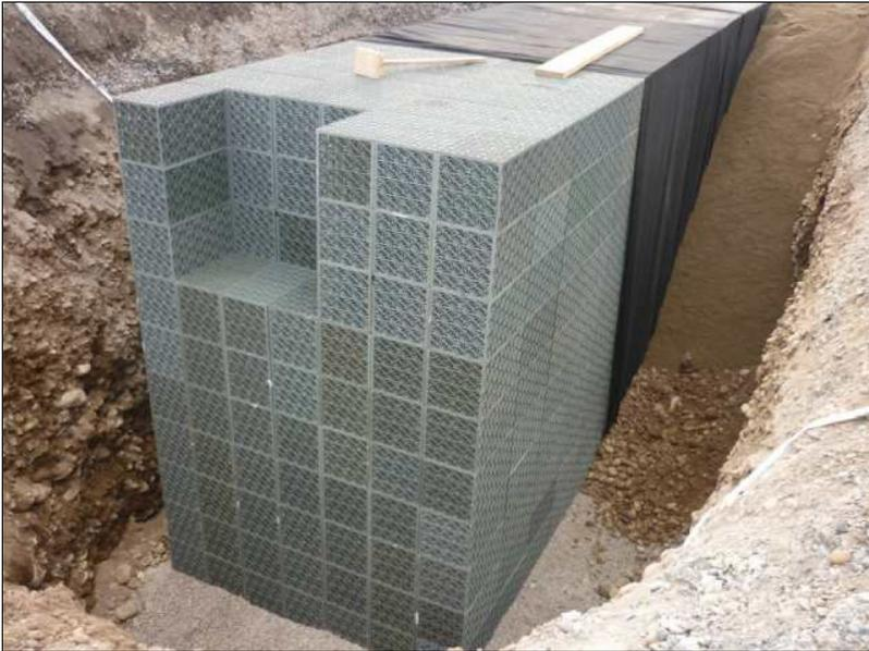
**The challenge:** The construction of HP Data Center involved a total catchment area (including roofs and ground surface) of 21,496 m<sup>2</sup>, for which HRI Consulting Engineers Ltd would design an infiltration trench that could store stormwater and infiltrate the required volume of water generated by a return period of 10 years in an area of vehicle traffic.
